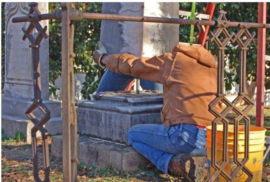
A 12 foot obelisk is being reset after drilling and insertion of a pin to prevent it from being easily toppled (photo in Chicora collections).
